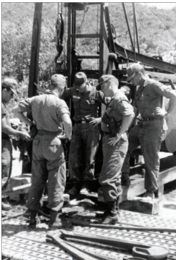
(Above) Capt. Ted Stroup, USA, with the 171st Well Drilling Detachment at Hon Tre Island, while commanding C Company, 864th Engineers. (Opposite) In the C Company prefabrication yard at Camp McDermott, Nha Trang.
