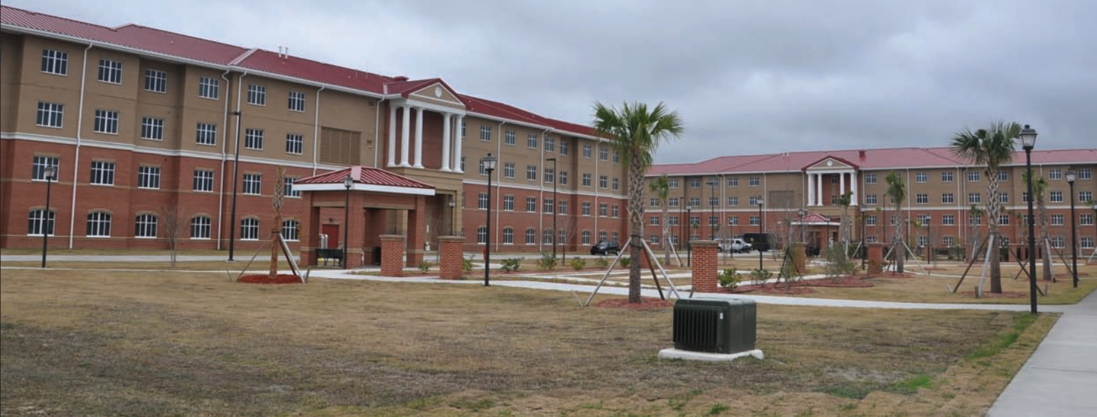
Construction on the $25.1 million Warrior in Transition barracks complex at Fort Stewart, Ga., was completed in 2012. USACE SAVANNAH DISTRICT PHOTO BY TRACY ROBILLARD
